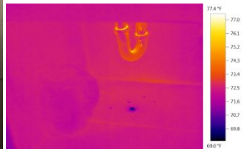
Bathroom 1: water on cabinet floor from leak at drain
