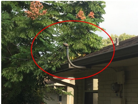
Rear: Foliage close to structure
