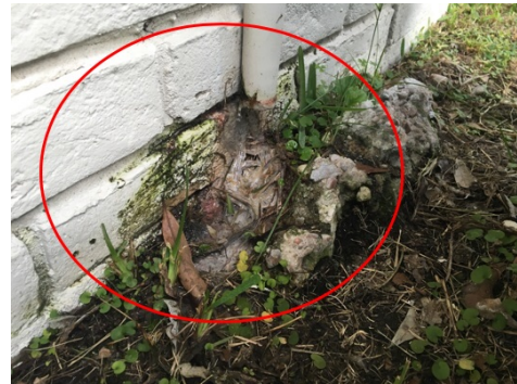
Primary condensate drain line draining on foundation and wall
