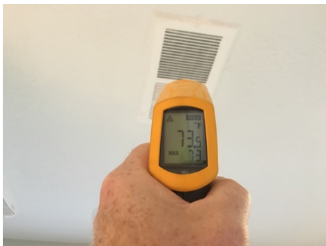
Temperature measured in bathroom 1
