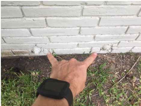
Right rear: cast iron drains
