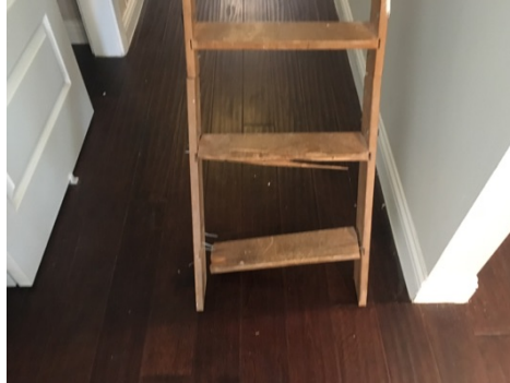
Pulldown stairs: Cracked steps
