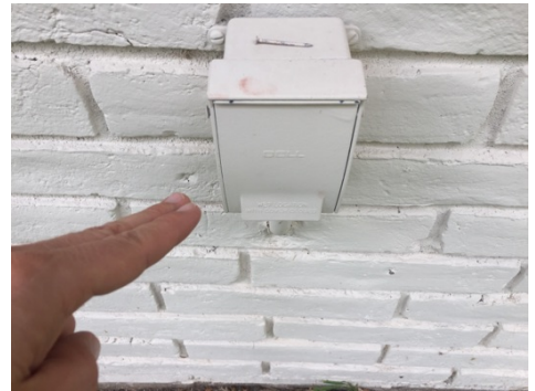
Exterior outlets: Bubble cover recommended
